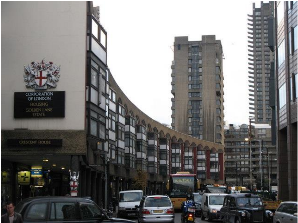
Crescent House with the Barbican Estate in the background (taken looking south down Goswell Road)
