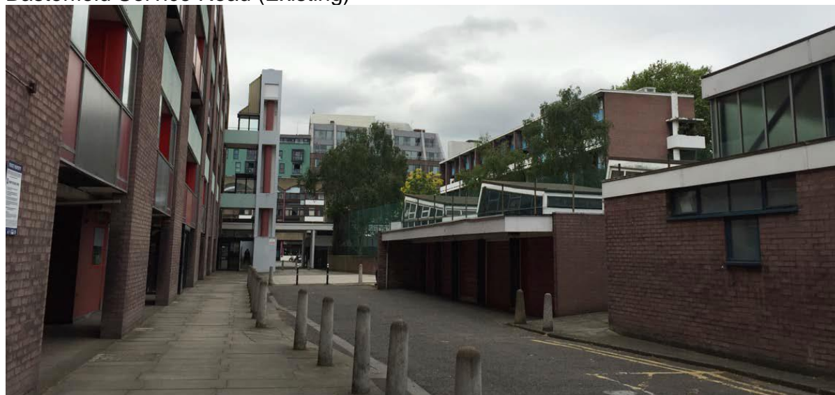
Basterfield Service Road (Existing)
