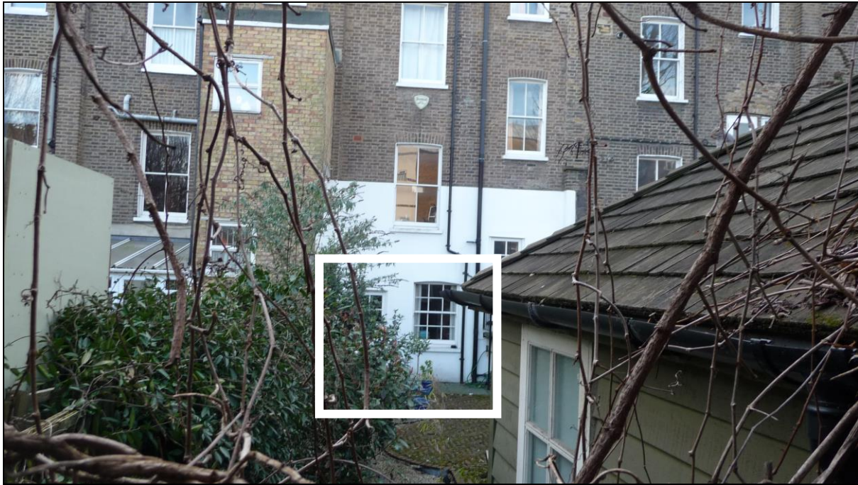
Fig. 28: Photo of the rear of No. 12 Packington Street. The room in question is lit by a window and glazed door (as outlined in white rectangle). Both window and door were taken into account in the daylight distribution analysis.
